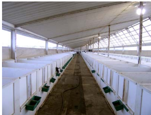
Figure 1. Interior view of a naturally ventilated calf barn with four rows of pens. There is a ridge opening above the translucent-panel roof to the south, adjustable curtain sidewalls, and individual calf pens surrounded by solid panels and a feeding opening in the front.
