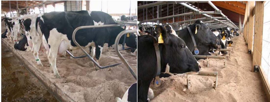
Figure 1. A remodeled stall (left) with sand on a concrete platform and a fiber glass bedding retainer, and new stalls (right) which are 10 feet long against the side wall to accommodate front lunge.
