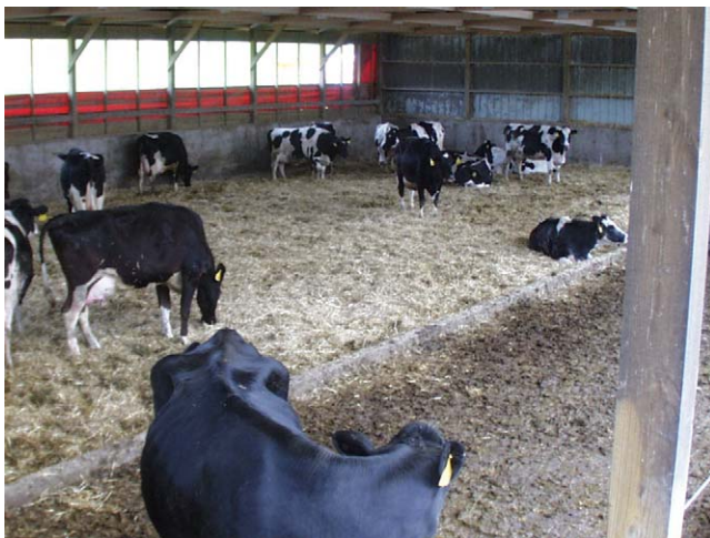
Fig. 2. A correctly designed, well ventilated, loose housed straw bedded pack area for dry cows, with a bedding retainer, wide access to the bedded area and a concrete apron in front of the feed bunk.
