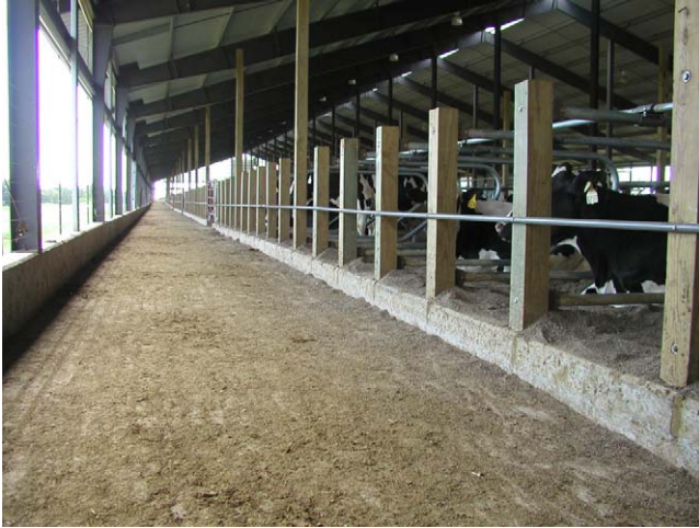
Fig. 3. A transfer alley used to move cows between pens in a well-managed transition cow facility. Although the front of the stalls are open, note the deterrent bar that is located too low to allow cows freedom to lunge forward in the stall.
