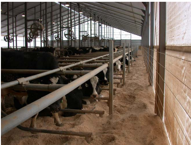
Fig. 6. An open front stall against a side wall, allowing uninhibited forward lunging of the head, free of obstruction. Dividers use a vertical mounting system at the bottom to avoid obstructing the lunge-and-bob movement of the head.
