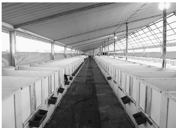
Fig. 1. Interior view of a naturally ventilated calf barn with four rows of pens. There is a ridge opening above the translucent-panel roof to the south, adjustable curtain sidewalls, and individual calf pens surrounded by solid panels and a feeding opening in the front.
