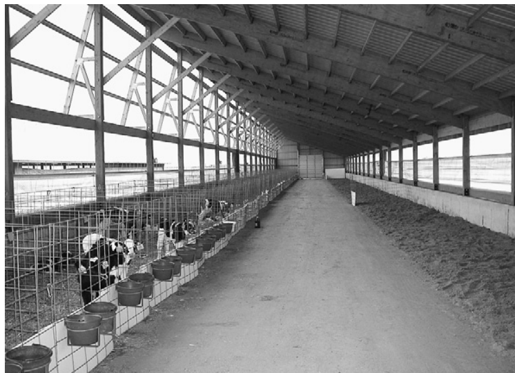
Fig. 2. Interior view of a naturally ventilated calf barn. The pens on the left are constructed of wire mesh panels, and the pens on the right side have been removed for cleaning.
